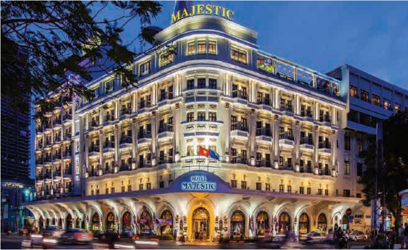
MAJESTIC HOTEL RENOVATION
