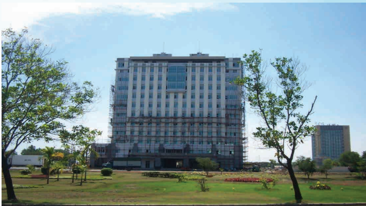
OFFICE BUILDING IN PHÚ MỸ HƯNG
