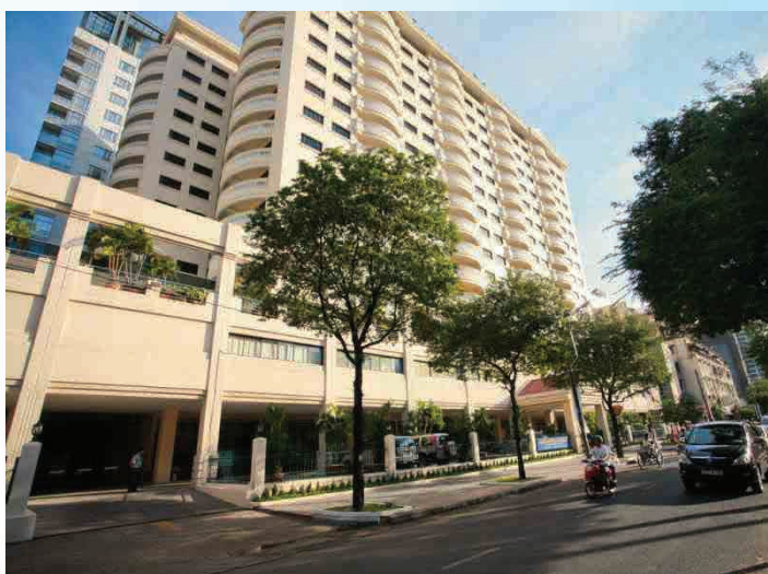
NORFOLK SERVICED APARTMENTS
